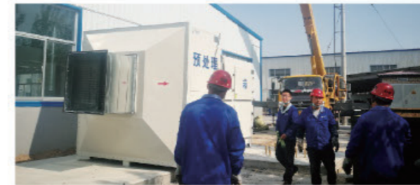
某军工车间 (过滤式除尘器) Anshan Qikai Chemical (Activated carbon adsorption chamber)
