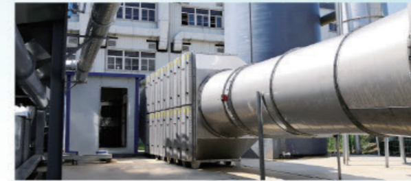
石家庄诚志永华 (活性炭吸附箱) Shijiazhuang Chengzhi Yonghua (Activated carbon adsorption chamber)
