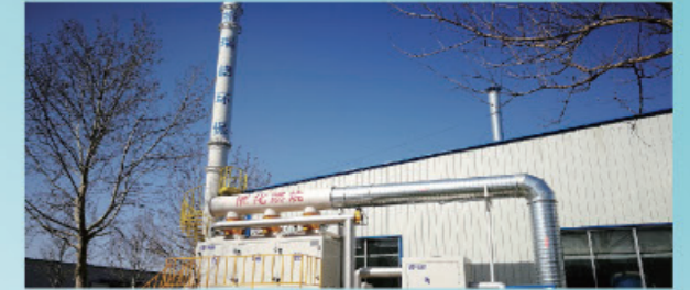
京东管业有限公司 (催化燃烧净化设备) Jingdong Tube Co.,Ltd (Catalytic combustion purification equipment)
